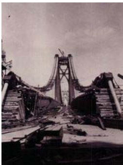
The Mid-Hudson Bridge under construction. (Photo: New York State Bridge Authority/Courtesy photo)
