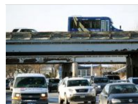
Northway lanes on new Exit 4 bridge to open
