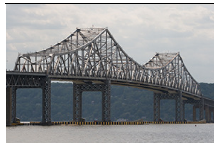
Tappan Zee Bridge
