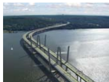
(Photo: Tappan Zee Constructors LLC and New York state Thruway Authority)
