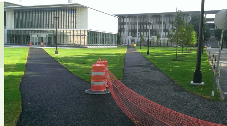
7,600SF Porous Asphalt Parking Lot and Walkways
