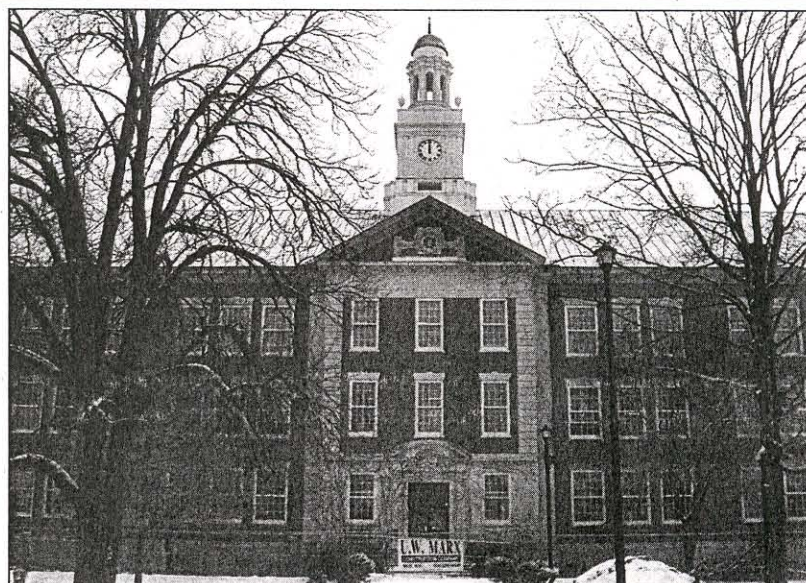
The finished tower.
