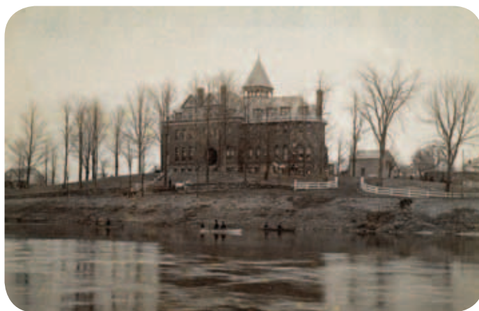
Former New Paltz Normal building along the banks of the Wallkill River.
