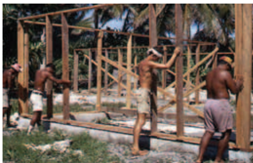
Doug Sheer '70 (Secondary Education/Social Studies) building a new co-op store and warehouse. His job was to be the advisor to the outer island co-operative.
